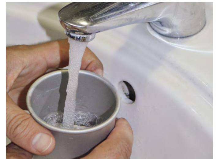
Faucet with aerator installed (air bubbles in water jet)
